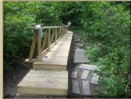
Here The Gang was working on replacing the longboards between the Jersey Bridge and the bike trail. The bridge is elevated and there are steps on either end.
